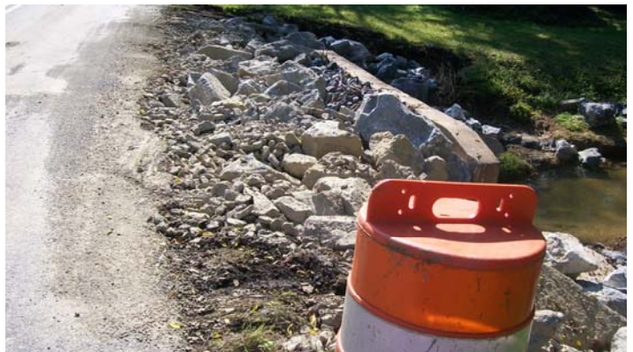
Emergency Stone Repair Work along Devonshire Hgts. Road
